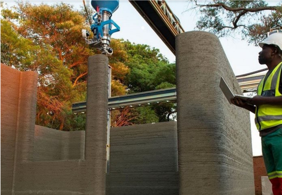
Malawi school being 3D printed. Source: Supplied
